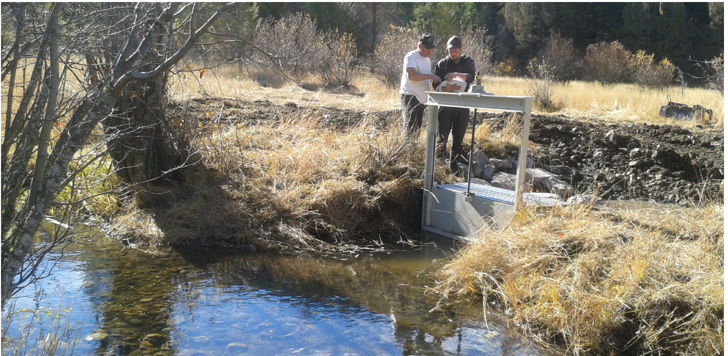
Irrigation headgate on Sauerkraut Creek
