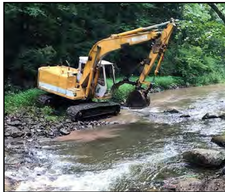
Wagner’s Dam (left); Instream rock structures were installed to reestablish the natural ecology of McMichael’s Creek, benefiting brook trout and other aquatic organisms (center)/Ben Turpin, Pohoqualine Fish Association; Completed restoration (right) will benefit not only recreational fly fishers, but also mitigate flooding in downstream communities/Ben Turpin, Pohoqualine Fish Association.
